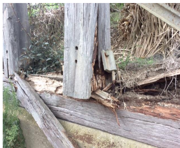
Bridge No. 263 on Swamp Road – damage to western piers and bearer
