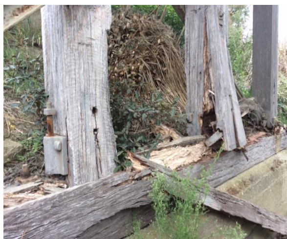
Bridge No. 263 on Swamp Road – damage to western piers and bearer
